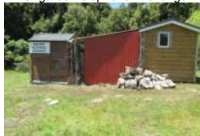
Ongarue Telephone Exchange
