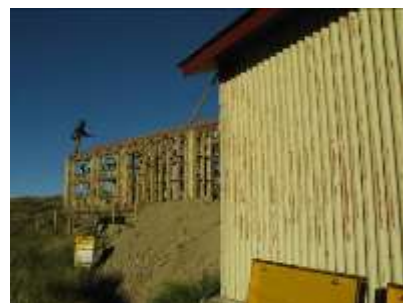
New Kime Hut construction
